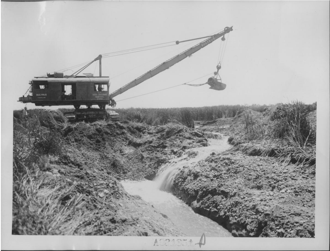
Figure 22 June 22, 1914 Electric Dredge excavating, Purdam Slough Drain on Lemp's Ranch." 108
