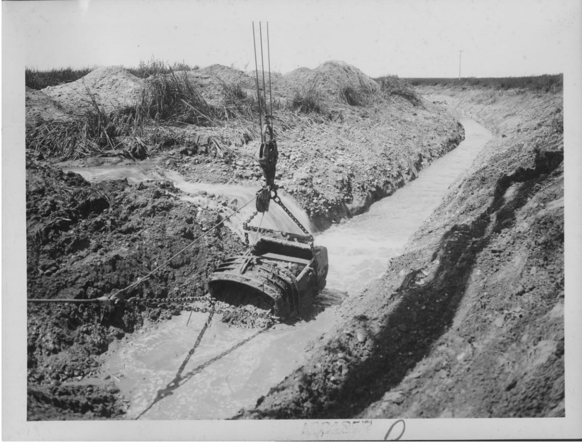
Figure 23 June 22, 1914 "Dredge bucket loading in hard cemented gravel on Purdam Slough Drain." 109
