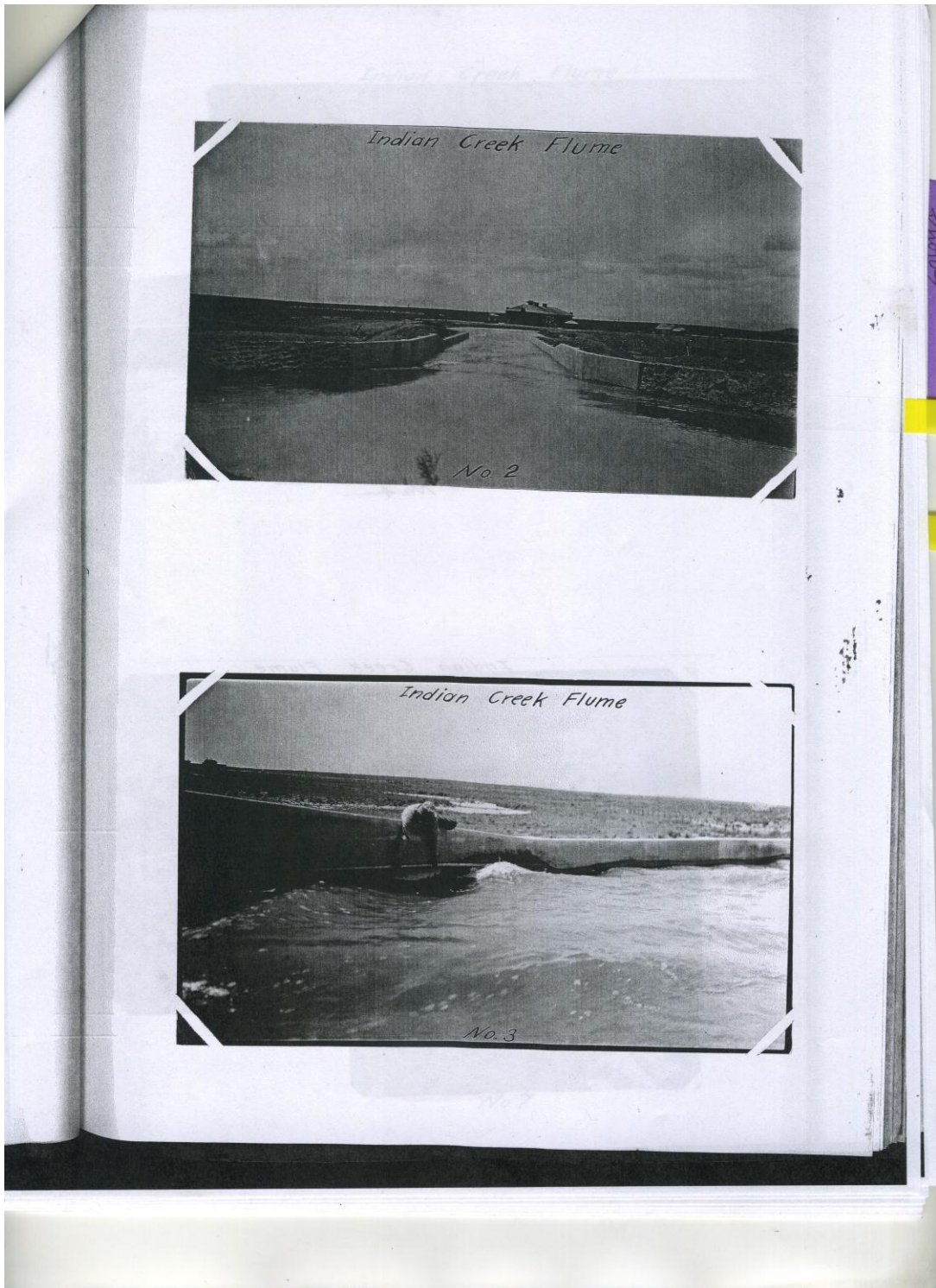
Figure 29 Indian Creek Flume 123
