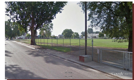
Left: In-pavement markers such as this were purchased by the City and should be used in crosswalks near Canyon Spring High School. Right: Extending the sidewalk facilities around the inlet box and tree allows for a continual pedestrian access route and thus, compliant with ADA by not forcing walkers into the street
