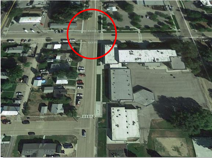
(Above) The Denver Street corridor is a parallel route to Chicago Avenue which can be busy with people and traffic. Drivers often use Denver as an alternative and have no real design prompts to slow travel speed. Adding stop controls at the 11th street intersection will reduce speeding traffic, highlight the presence of walking students, and minimize conflicts at the intersection.
