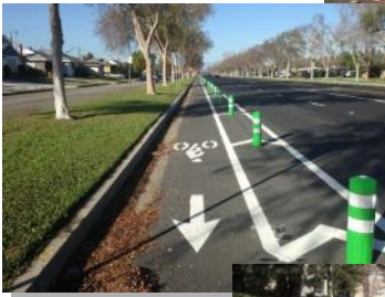
Buffered bike lanes can take many forms and use several tools to separate the bike lane from the travel or parking lane.
