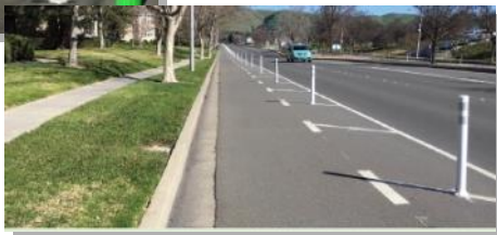
Buffered bike lanes can take many forms and use several tools to separate the bike lane from the travel or parking lane.
