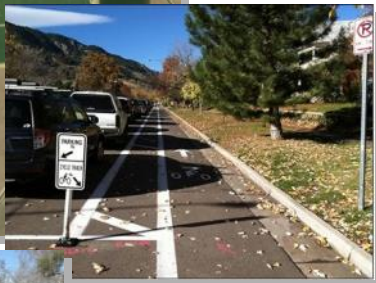
Buffered bike lanes can take many forms and use several tools to separate the bike lane from the travel or parking lane.
