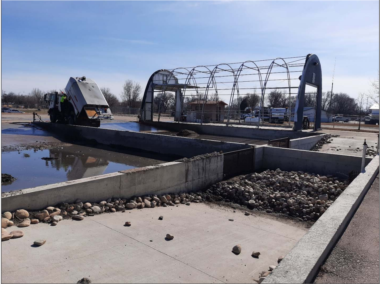
Figure 4. Wash Rack Outdoor Wash Bays
