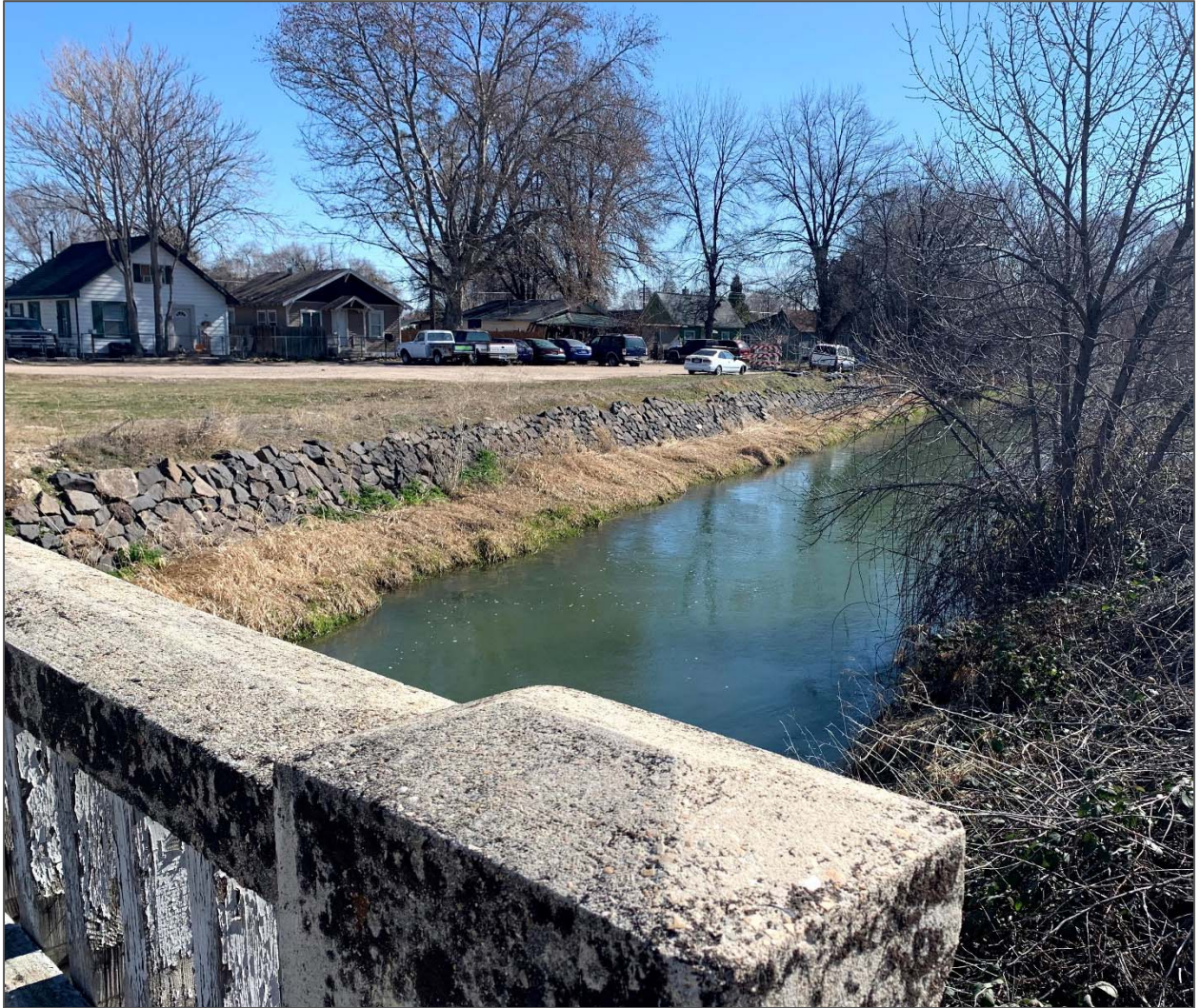
Indian Creek at the 12 th Avenue Outfall, Downtown Caldwell
