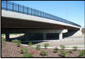
New Interchange at I-84 Exit 29 at Hwy. 20/26
