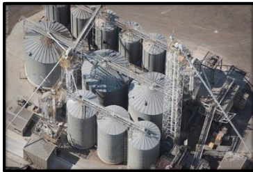
Above: Grain Silos in Caldwell.
