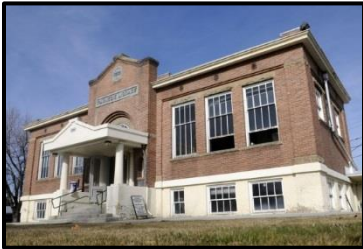
Below: Carnegie Library; the Current Home of the Caldwell Veteran's Council.
