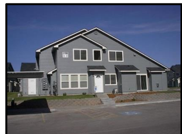
Below: Four-plexes, apartment complexes and manufactured home parks are commonly found in high density zones. Lower density uses may be permitted.
