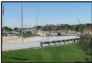
Above: Exit 29 Interchange.
