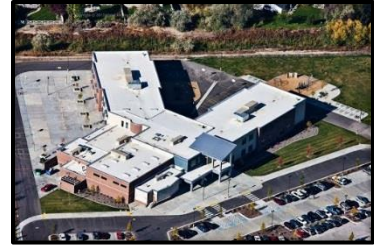
Above: Washington Elementary School, Caldwell School District #132.
