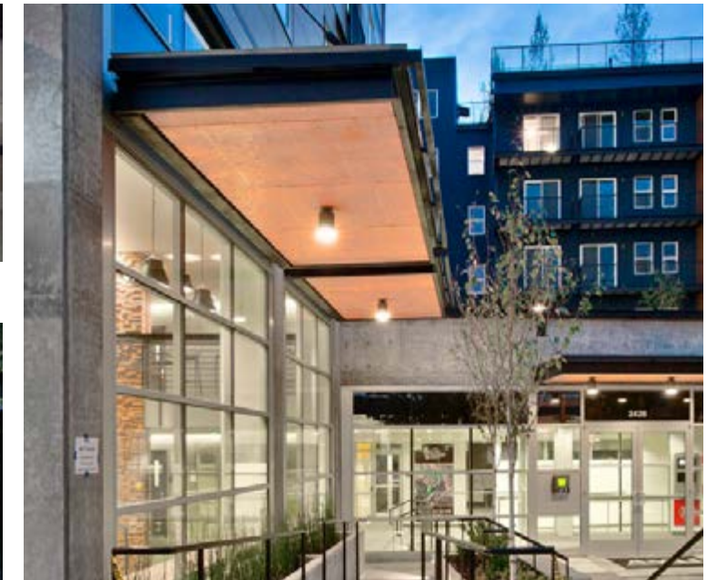
Kit #3 Steel frame canopy with material unique to retailer at underside
