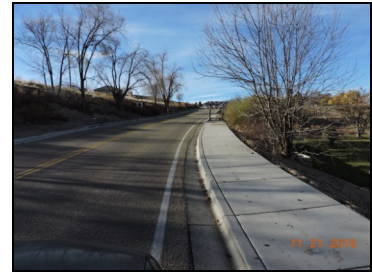
Above: Sidewalk on Marble Front Road.
