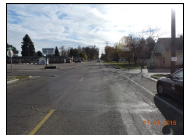
Above: Kimball Avenue at Ash Street.
