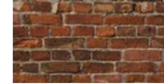
Restore Existing Brick
